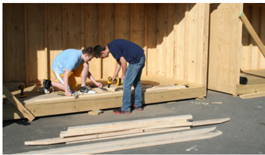
From left, Connor McGrath and Ricci Shenck work on building a truss in the dugout
