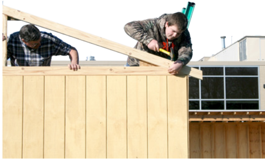
Kyle Ierlan, on right, nails a truss to the shed while teacher Tim Rogers supervises
